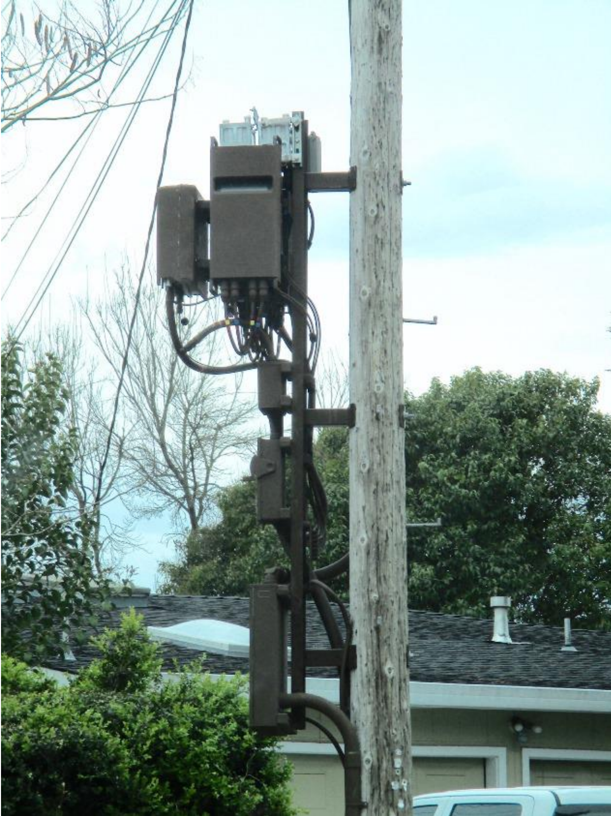
Unfinished 5G Cell Tower Being Built in Santa Rosa, CA - mummyanglais.wordpress.com
